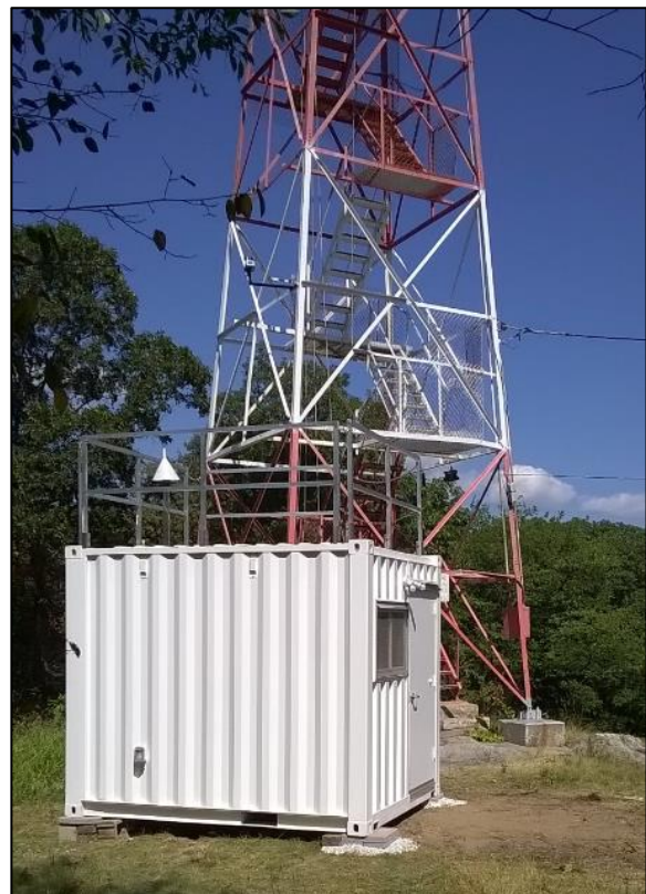
Figure 2-1 Ramapo Air Monitoring Station
